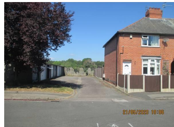
View of no. 83 to the right and site facing west
