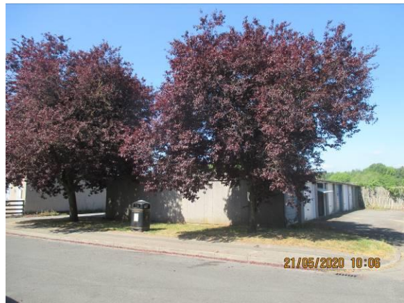
View of site facing west
