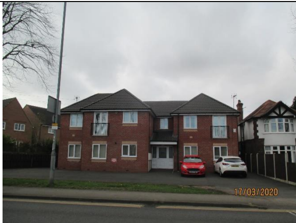
Front elevation to the site
