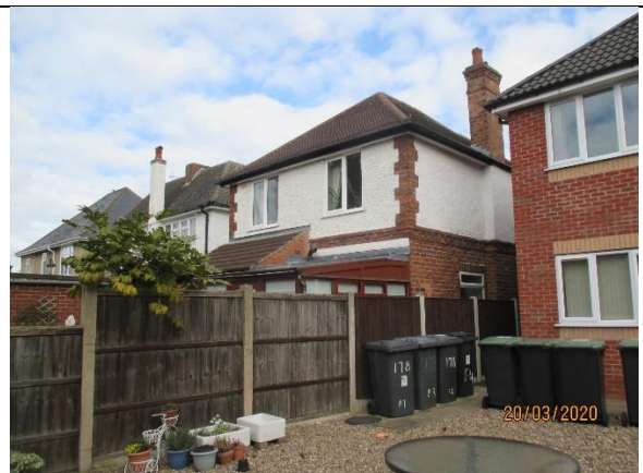
Rear of 176 Bye Pass Road
